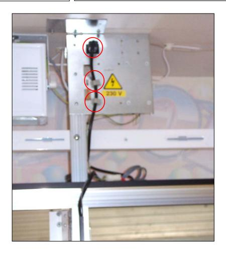
• Connect the crane to the current network (outside the head).
