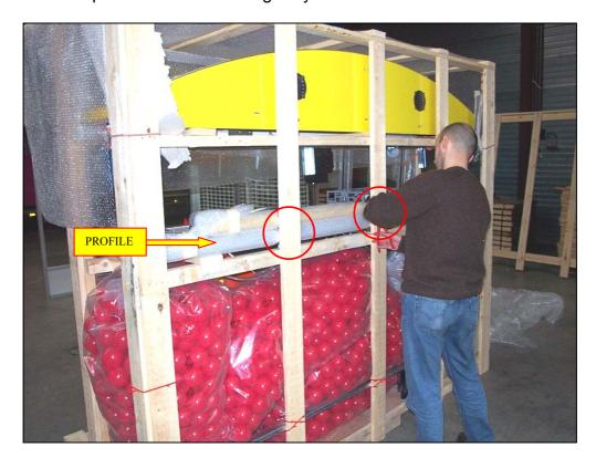
• Unwrap the longest pack and position the partitioning profile (= profile with 2x two pins) between the two sides (see drawing). Attach this profile in the provided holes with a rubber hammer.
